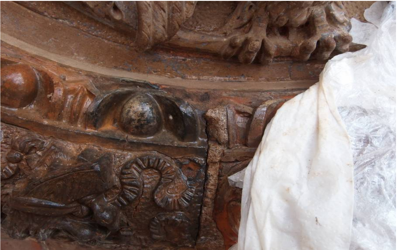
Different coloured lime mortars on terracotta after being covered with damp paper towels and clingfilm
