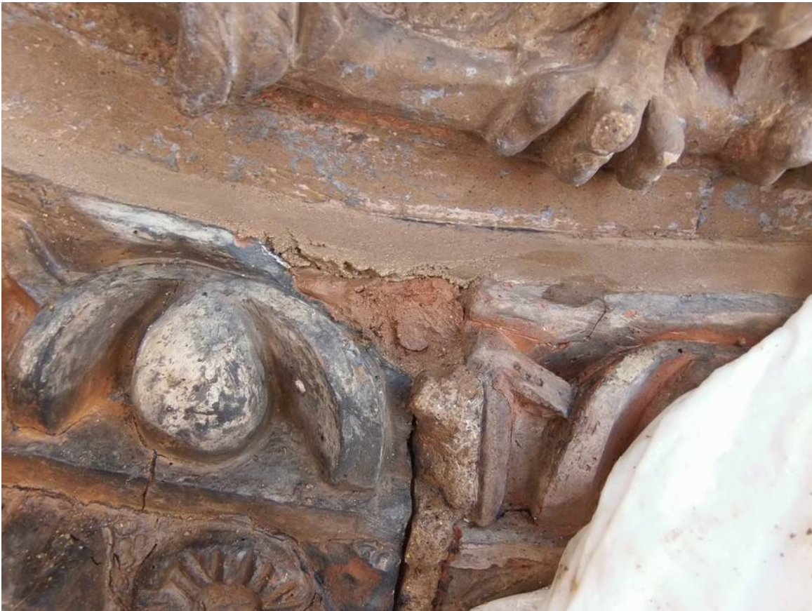
Applying different coloured lime mortars to terracotta
