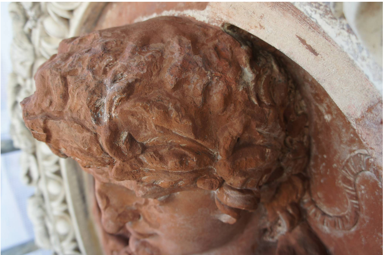
Terracotta head after grouting with Ledan TB1
